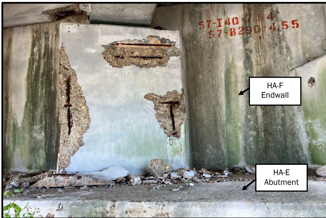
Photo 5: View of HA-E and HA-F from the southeast end of the bridge.
