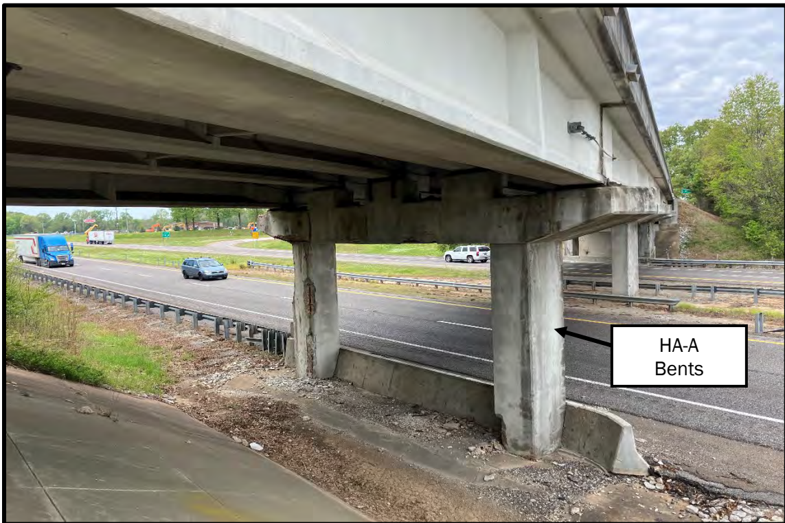
Photo 2: View of HA-A from the southeast portion of the bridge.
